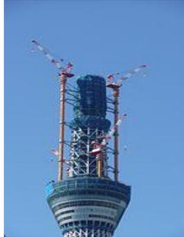
Generally a type of tower crane, these cranes, also called self-assembling, jack-up, or "kangaroo" cranes, lift themselves from the ground or lift an upper, telescoping section using jacks, allowing the next section of the tower to be inserted at ground level or lifted into place by the partially erected crane itself. They can thus be assembled without outside help, and can grow together with the building or structure they are erecting.
