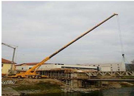
A crane mounted on a truck carrier provides the mobility for this type of crane. This crane has two parts: the carrier often referred to as the Lower, and the lifting component which includes
