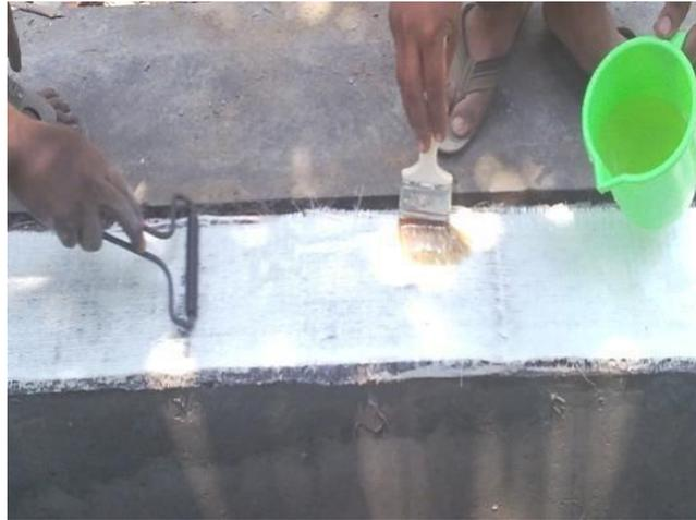
**Fig. 5 GFRP lamination in progress**
