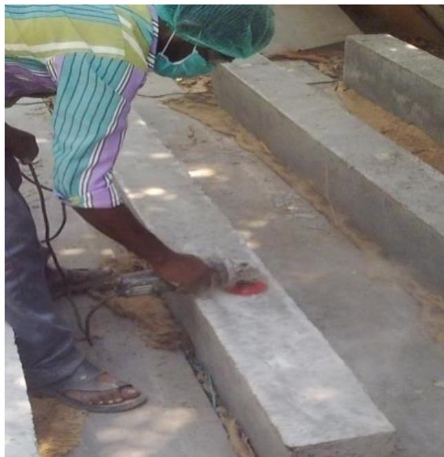
**Fig.4 Surface grinding in progress**
